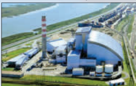
Portugal Solid Waste Investment Plan – EGF Group waste treatment infrastructure
